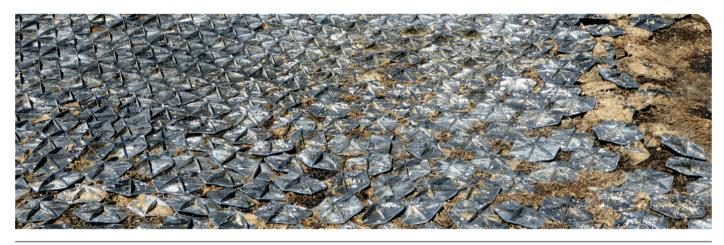
Figure 40. Round liquid manure storage with floating permanent cover comprised of plastic hexagon discs (L2).
