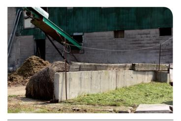
**Figure 34.** An uncovered solid *manure storage* with covered liquid runoff storage (V4).
