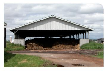
Figure 32. Covered solid *manure storage* (V2) with slatted walls.
