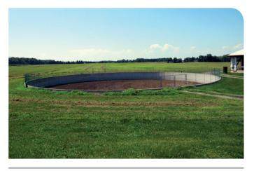
**Figure 41.** In-ground, uncovered, vertical wall liquid *manure storage* (M1).
