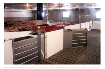
**Figure 35.** Slatted floor of barn for liquid *manure* storage under the barn (V5).
