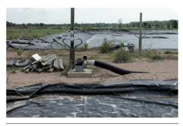
**Figure 36.** Tight-fitting negative pressure tarp for liquid earthen *manure storage* (V6).
