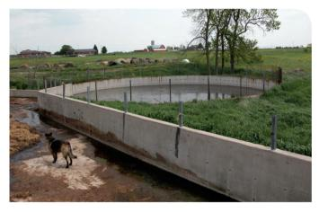
**Figure 39.** A solid, uncovered outdoor storage with uncovered liquid runoff storage (L1).
