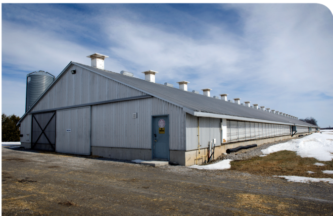
Figure 26. Exterior of a turkey barn.
