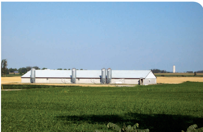
Figure 14. Exterior of a finishing swine barn with liquid manure storage under the barn.
