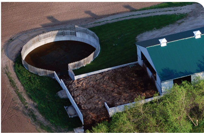
Figure 38. Uncovered liquid runoff storage (L1).
