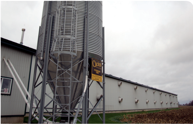
Figure 16. Exterior of a chicken broiler barn.*
