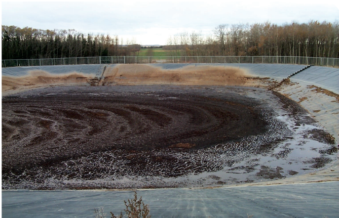
Figure 44. An earthen manure storage ; note the sloped sides and no cover (H1).
