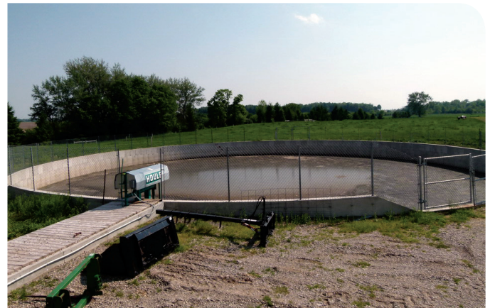
Figure 42. An above-grade, uncovered, vertical wall liquid manure storage and clean-out access ramp (M1).
