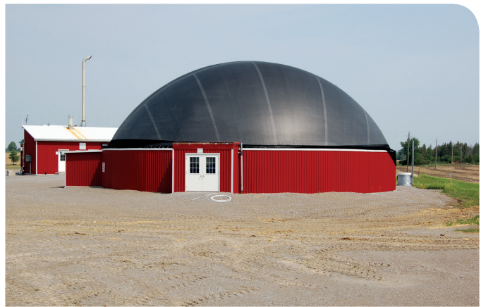
Figure 37. Raised base of liquid storage with tightly-sealed inflatable dome cover visible (V6).
