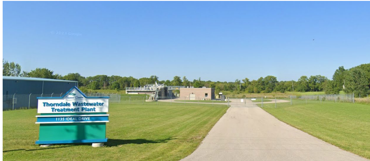
Existing Thorndale WWTP (Google Streetview, 2023)
