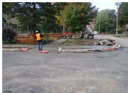
Typical Installation of new sidewalks and curbs
