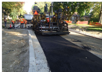
Typical Installation of new asphalt
