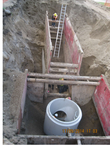
Typical Installation of new sewer
