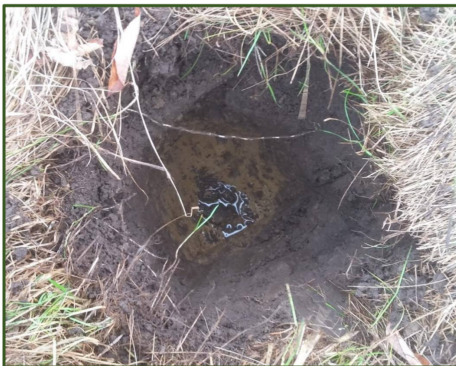
Photo 8: Typical Test Pit Facing North
