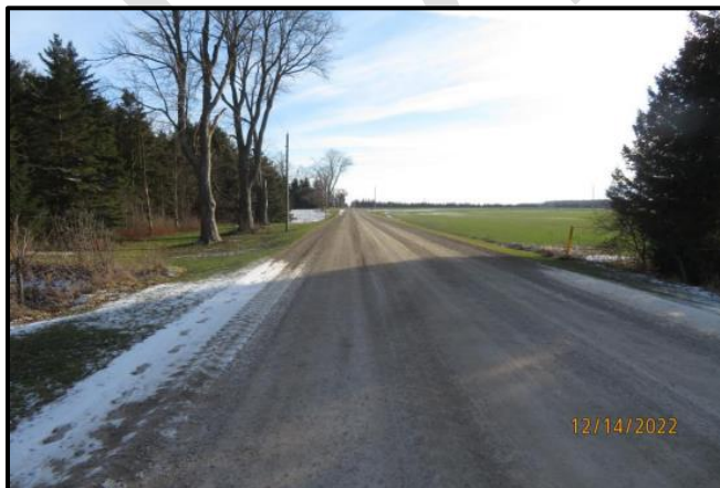
Cherry Hill Road Culvert - No. 134 (BCI = 71 Good)
