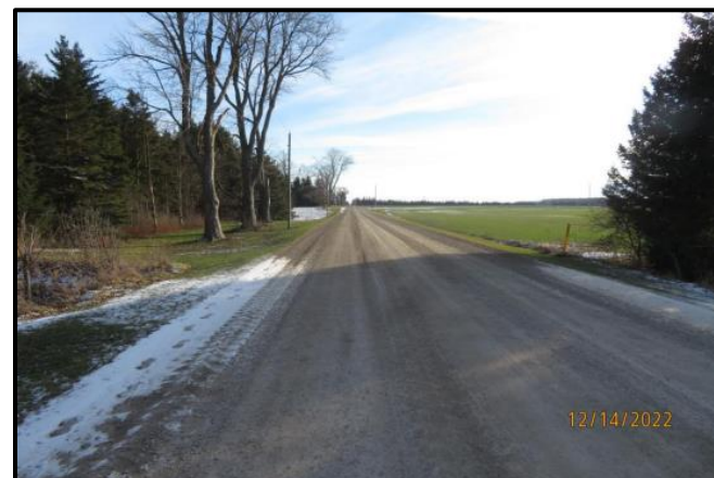
Cherry Hill Road Culvert - No. 134 (BCI = 71 Good)
