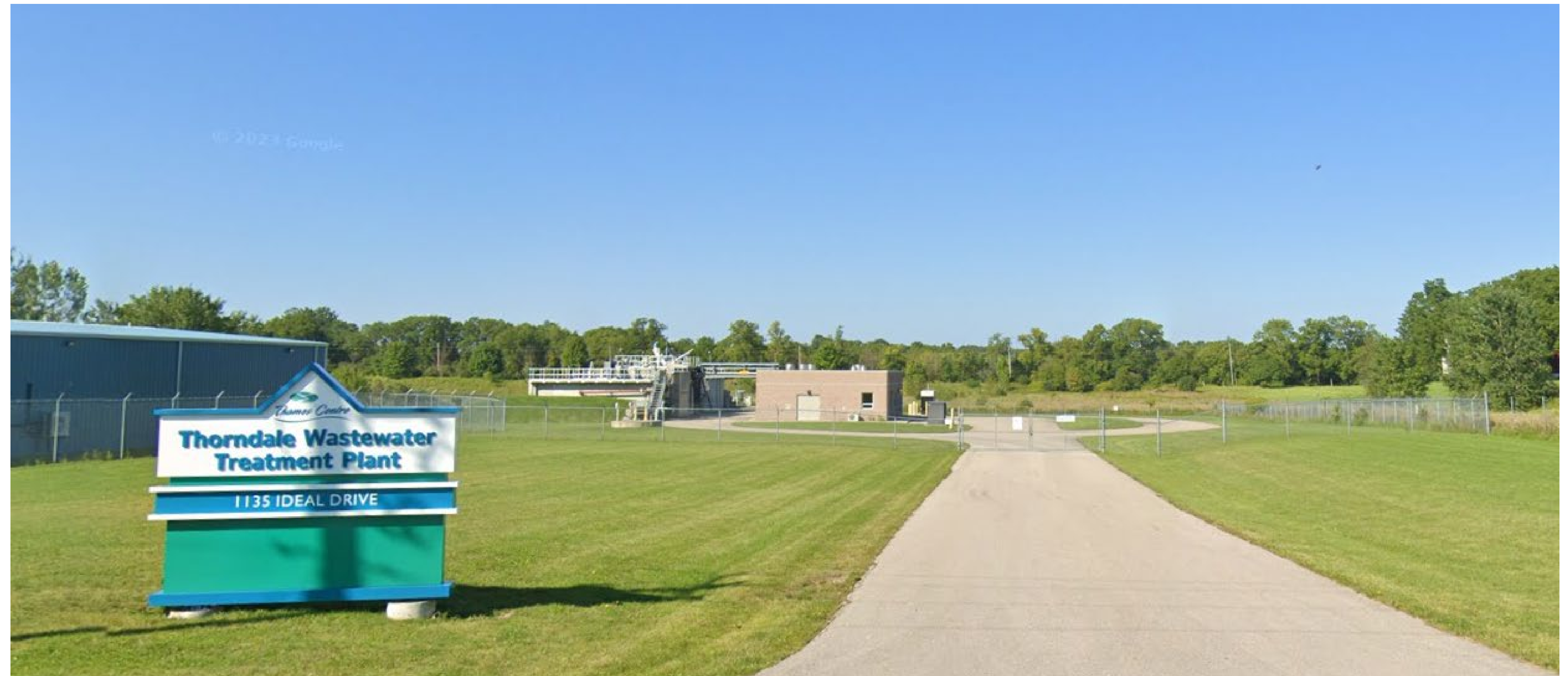
Existing Thorndale WWTP (Google Streetview, 2023)
